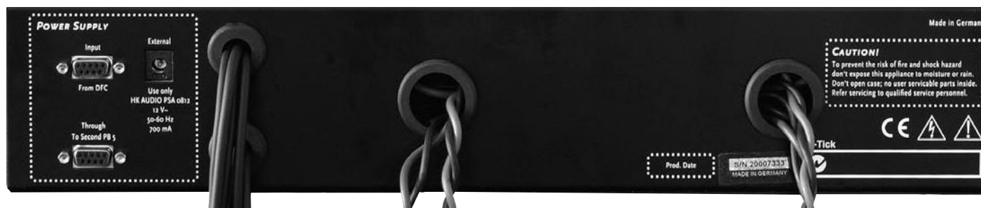
Figure 2: PB 5 rear view with patch cables
