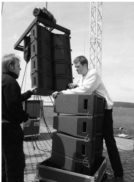
Figure 16: Hoisting the top four COHEDRA® mid/high enclosures
