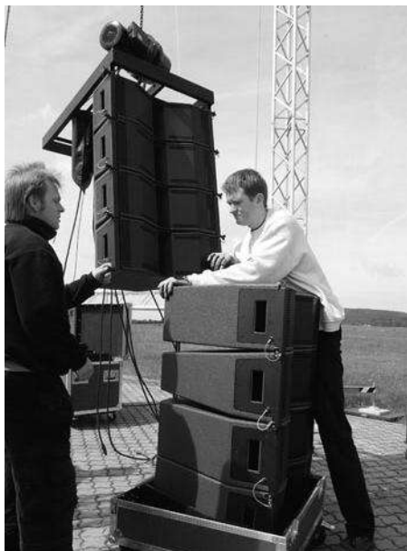
Figure 16: Hoisting the top four COHEDRA® mid/high enclosures
